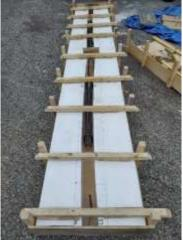
Fig. 4 Forms for curved UHPC beams
